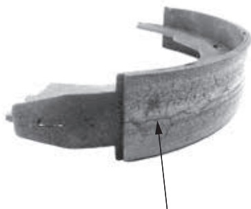
Acceptable Hairline Cracks
